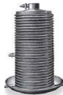
1879 – Counter flow external surface cooler
