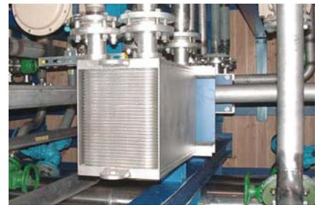
SIGMAWIG ST12 tempering of chemical reactor thermo-oil / ethylenglycol
