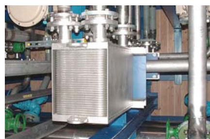
SIGMAWIG ST12 tempering of chemical reactor thermo-oil / ethylenglycol
